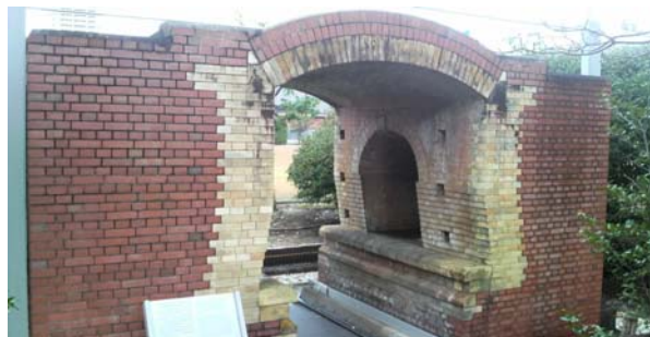
Figure 2. Cross section of a Harrop type kiln owned by NGK Insulators, Ltd. Photo by the author
