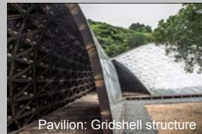
Pavilion: Gridshell structure
